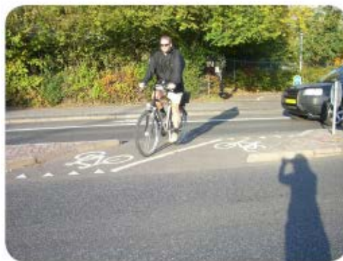
Medians on bicycle boulevards can provide space for a bicyclist to wait.
